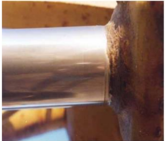
No pitting or corrosion after 1500 Hrs
